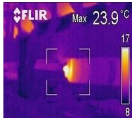
Bottom idler normal operating conditions.
