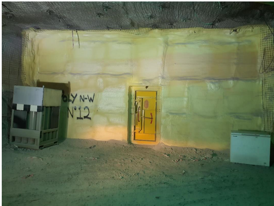
4(c) – A Residual Air Sealed Void with Emergency Bottled Oxygen Supply
